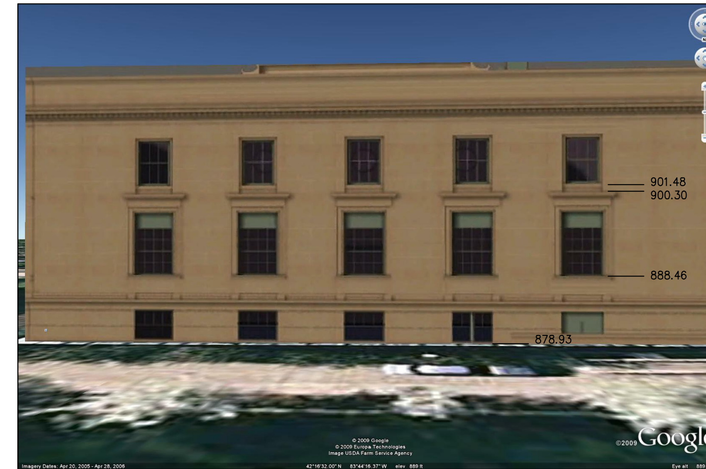
NORTH BUILDING FACE:
